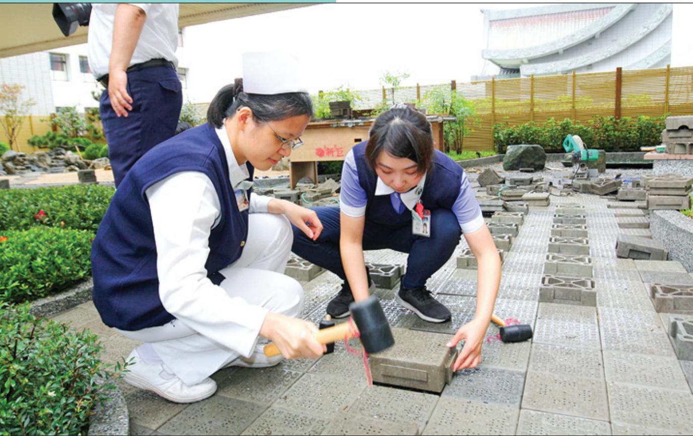
▲ A Filipino inventor volunteering for the Tzu Chi Foundation in Taiwan devised a way to turn the non-recyclable plastic layer in paper boxes and cups into floor tiles.
